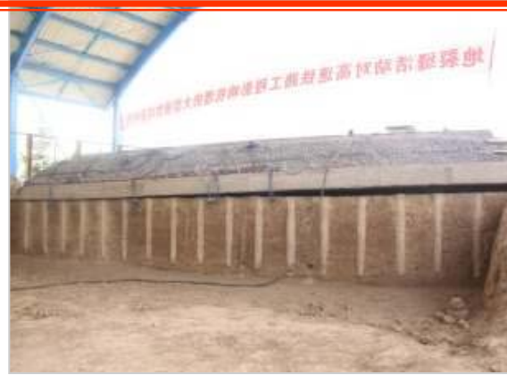
Cavity of piles
