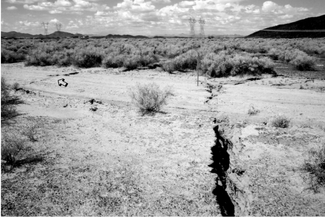
Figure 5. En echelon section of earth fissure crossing Baseline Road, looking NW. Fissure is 6-12 inches wide here. Second earth fissure crosses road at far left (arrow).
