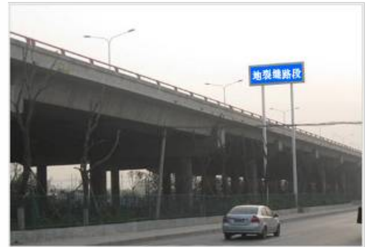
The test section of express loop highway
